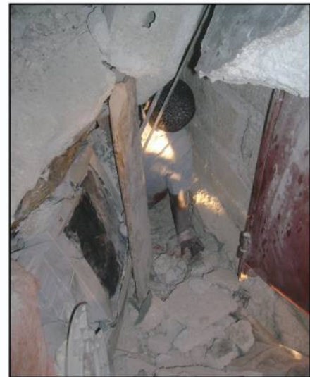
Makeshift shoring was used to rescue the boy, who was trapped in a triangular void space less than two feet wide.
